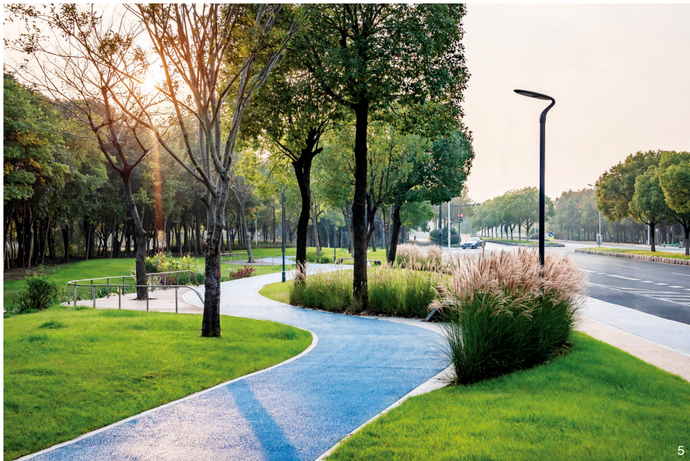
5 透水铺装实现道路雨水的自然下渗 Natural infiltration of road rainwater realized through permeable pavement
